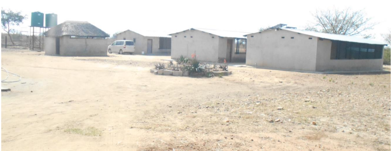
KITCHEN, WATER TANKS, AND FOWL RUNS FOR THE SKILLS CENTRE
